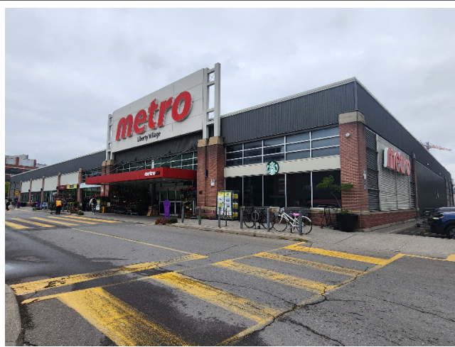
① Description: Building overview.
