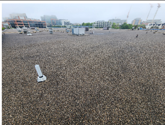
③ Description: Overview of roof area 2.0 (main roof level).
