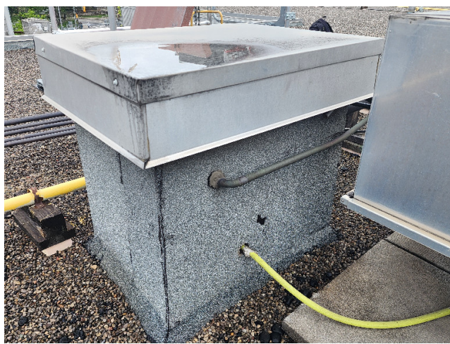
17 Description: Opening on the doghouse.
