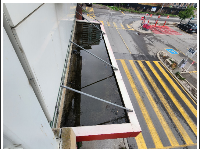
② Description: Overview of roof area 1.0.
