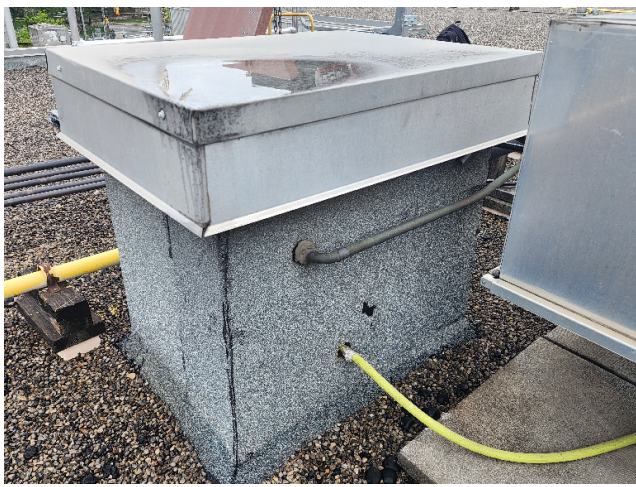
17 Description: Opening on the doghouse.
