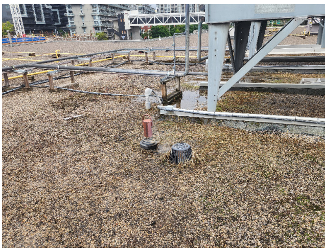
19 Description: Overview of large amounts of organic debris around the roof drain.
