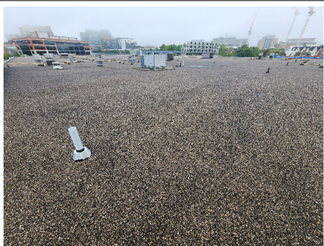
③ Description: Overview of roof area 2.0 (main roof level).
