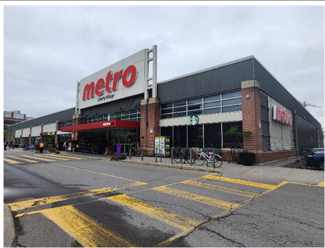
① Description: Building overview.
